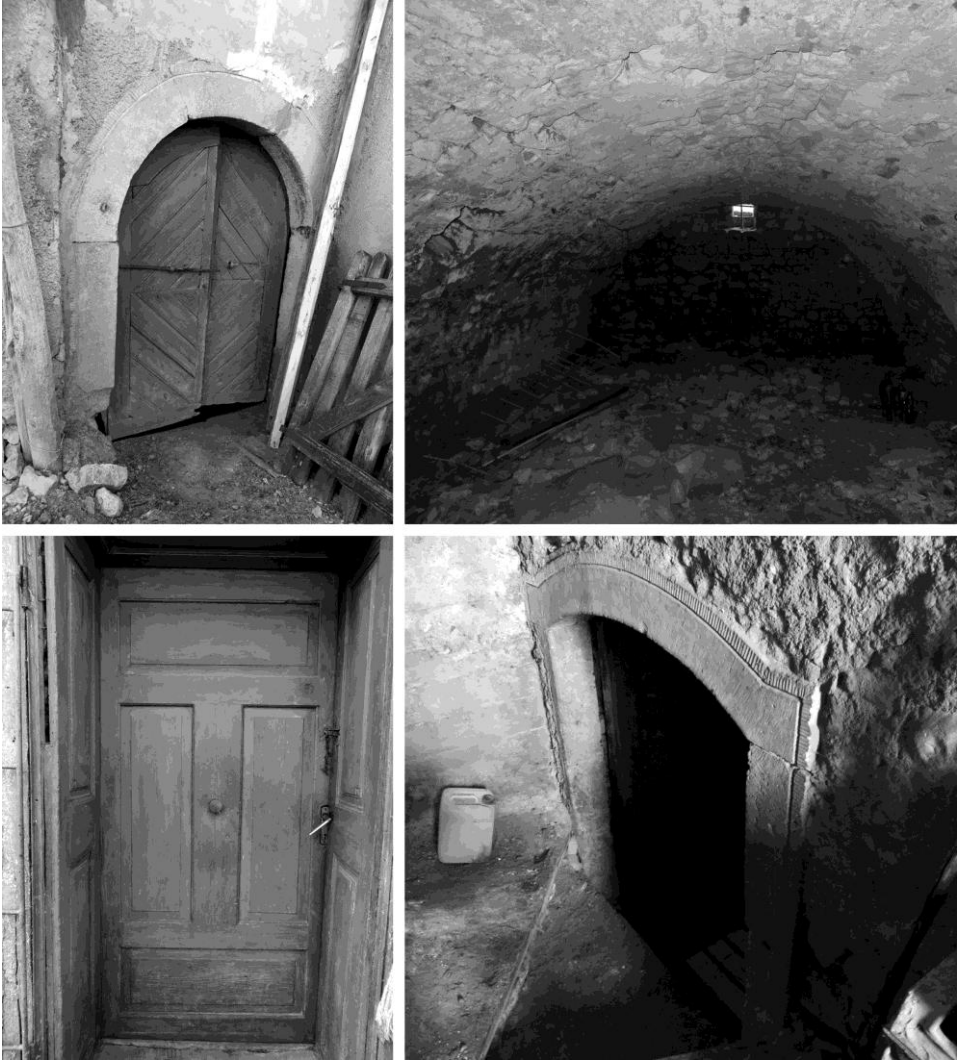
Fig. 8 Details of the former Fileki manor house in Suceagu: a - reused Baroque frame, the current upper entrance to the cellar; b - one of the still preserved rooms of the cellar; c - door preserved in situ, dating from the late 18 th century, early 19 th century; d - Baroque frame preserved in situ, the current lower entrance to the cellar. [The authors' archive, 2021]
