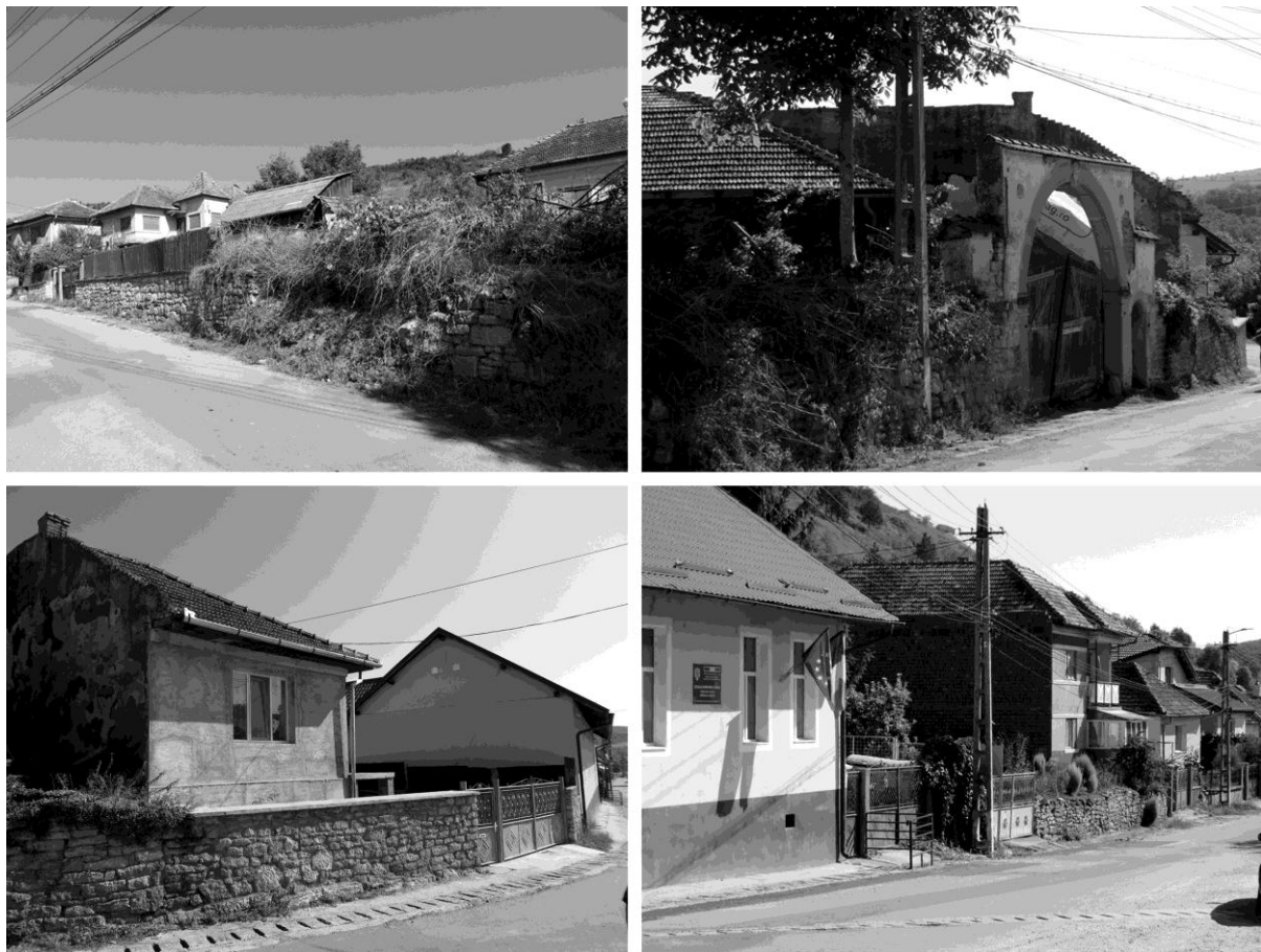
Fig. 6 Fragments of the precinct wall, including the Baroque gate, belonging to Sándor Fileki's former manor house in Suceagu. The last alterations are relatively recent. [The authors' archive, 2021]
